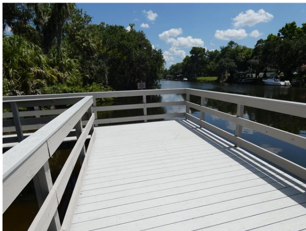
Dock Deck Boards/Railings
