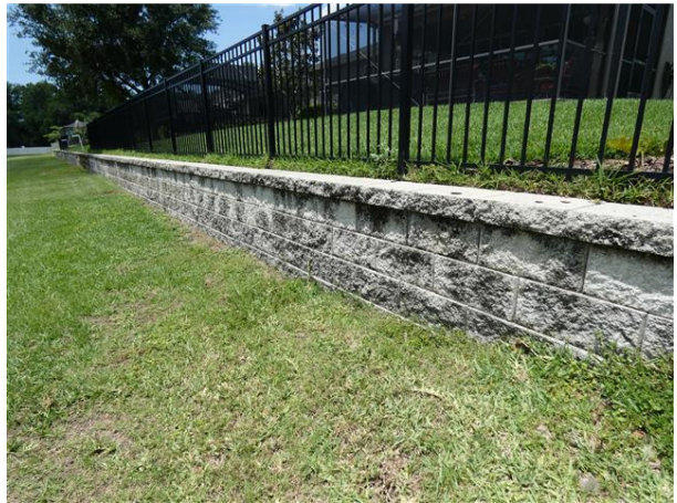
Retaining Walls Masonry
