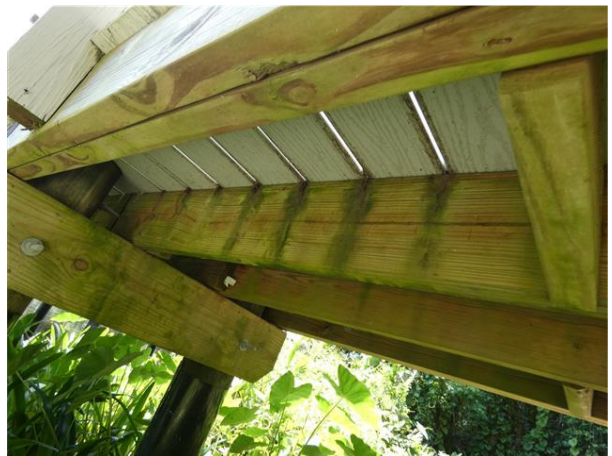
Dock Frame and Pilings
